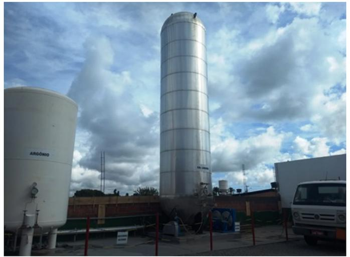
Foto 02 - Tanques de armazenamento de Argônio (à esquerda) e CO<sub>2</sub> (à direita).
