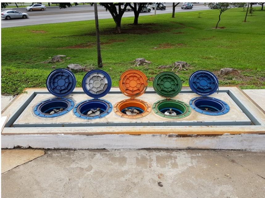
**Foto 07** - Descarga selada a distância, sem resíduos de combustível
